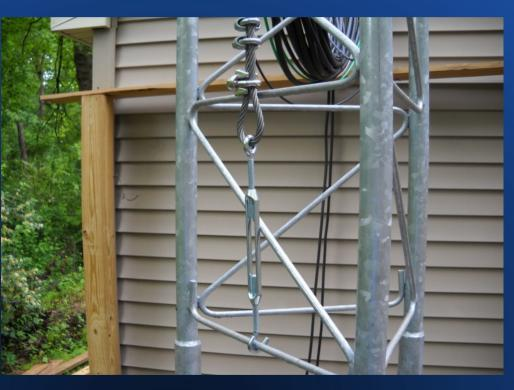
Secure at top and Adjustable at bottom
